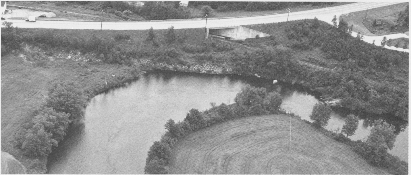
Two sections of earthfill dike totalling 657 feet help protect the farmlands of Coos County Institution in West Stewartstown from high velocity flooding and soil erosion. The Corps-built sections of dike replace segments of privately-built dike weakened during heavy flooding in 1973 and 1974. Pictured above is the 500-foot-long northerly dike segment at a bend in the Connecticut River.
