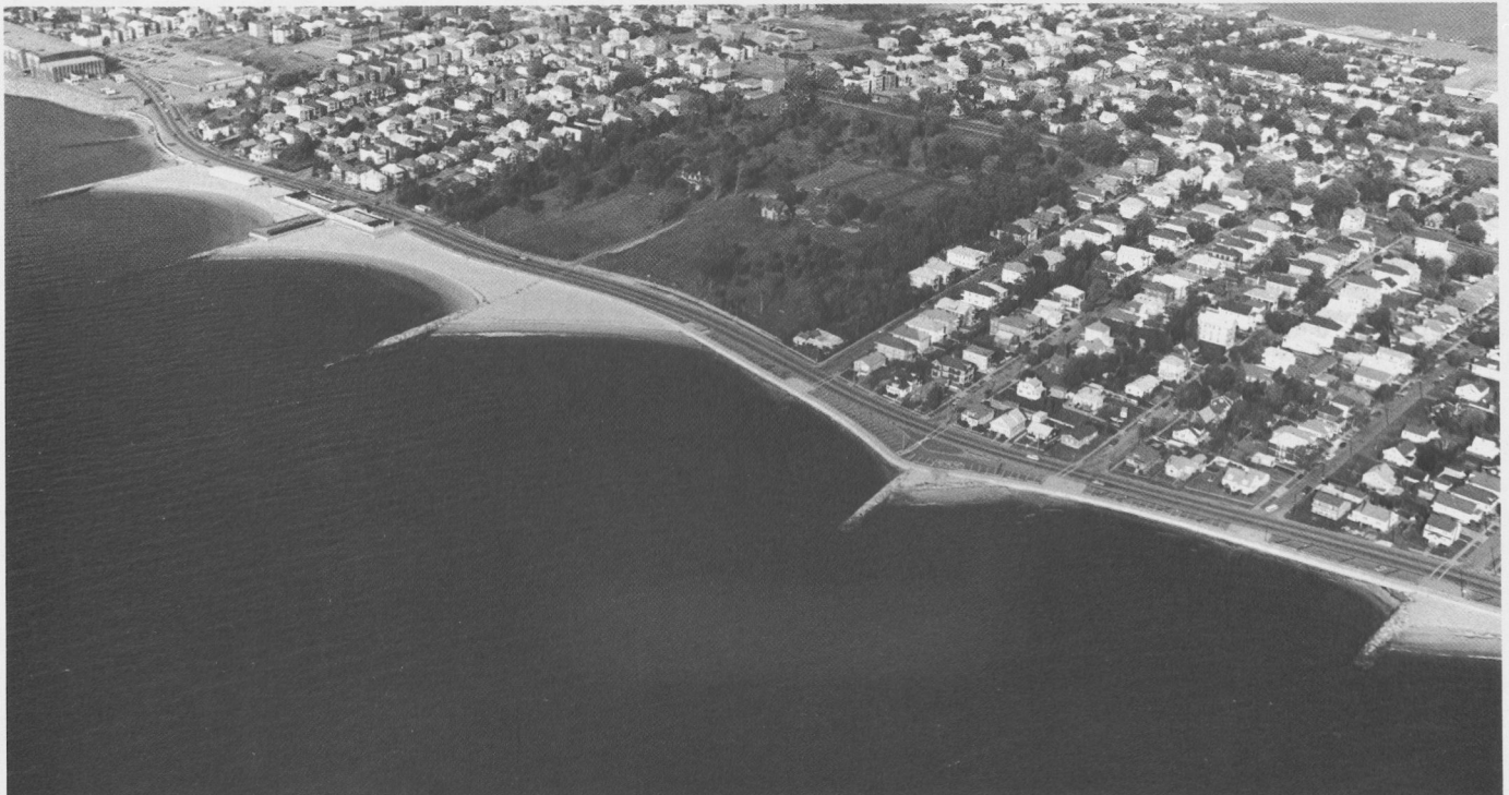
Groins help preserve New England's fragile shores and beaches that are subject to strong winds and waves. These Corps-built groins, at Clark Point in New Bedford, Massachusetts, retard erosion and help to maintain the stability of the shore.
