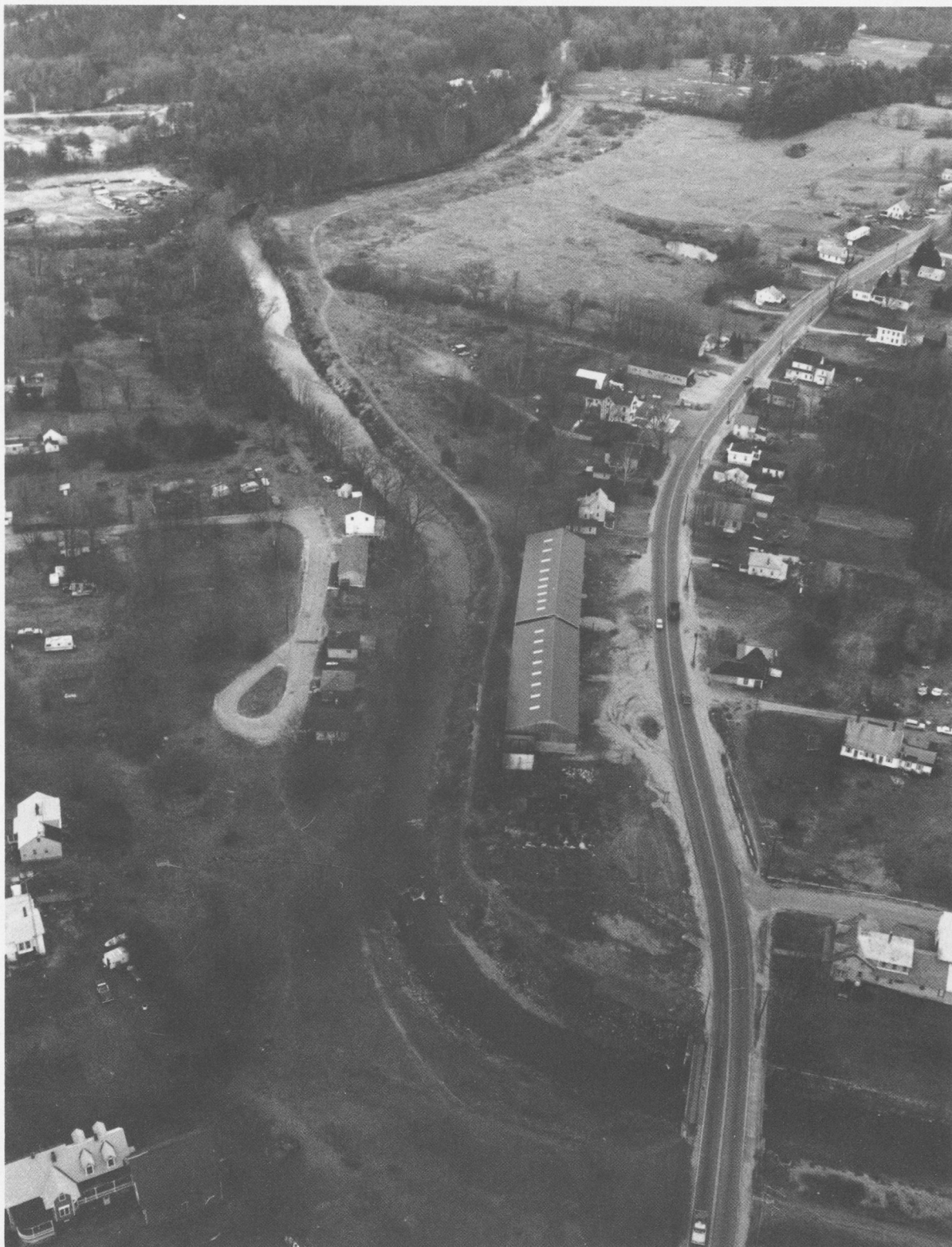
The lower half of the Cocheco River Local Protection Project included widening and deepening 4000 feet of the river, beginning at the South Main Street Bridge (lower right).
