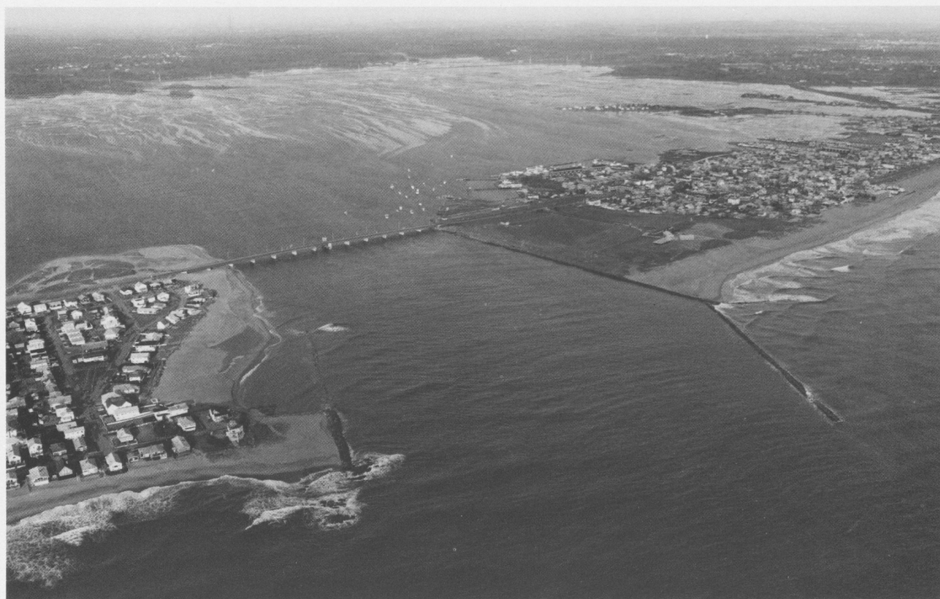
The entrance to Hampton Harbor separates Seabrook (left) and Hampton Beaches. The Corps constructed a channel through the entrance and extended and raised the stone jetties on either side.
