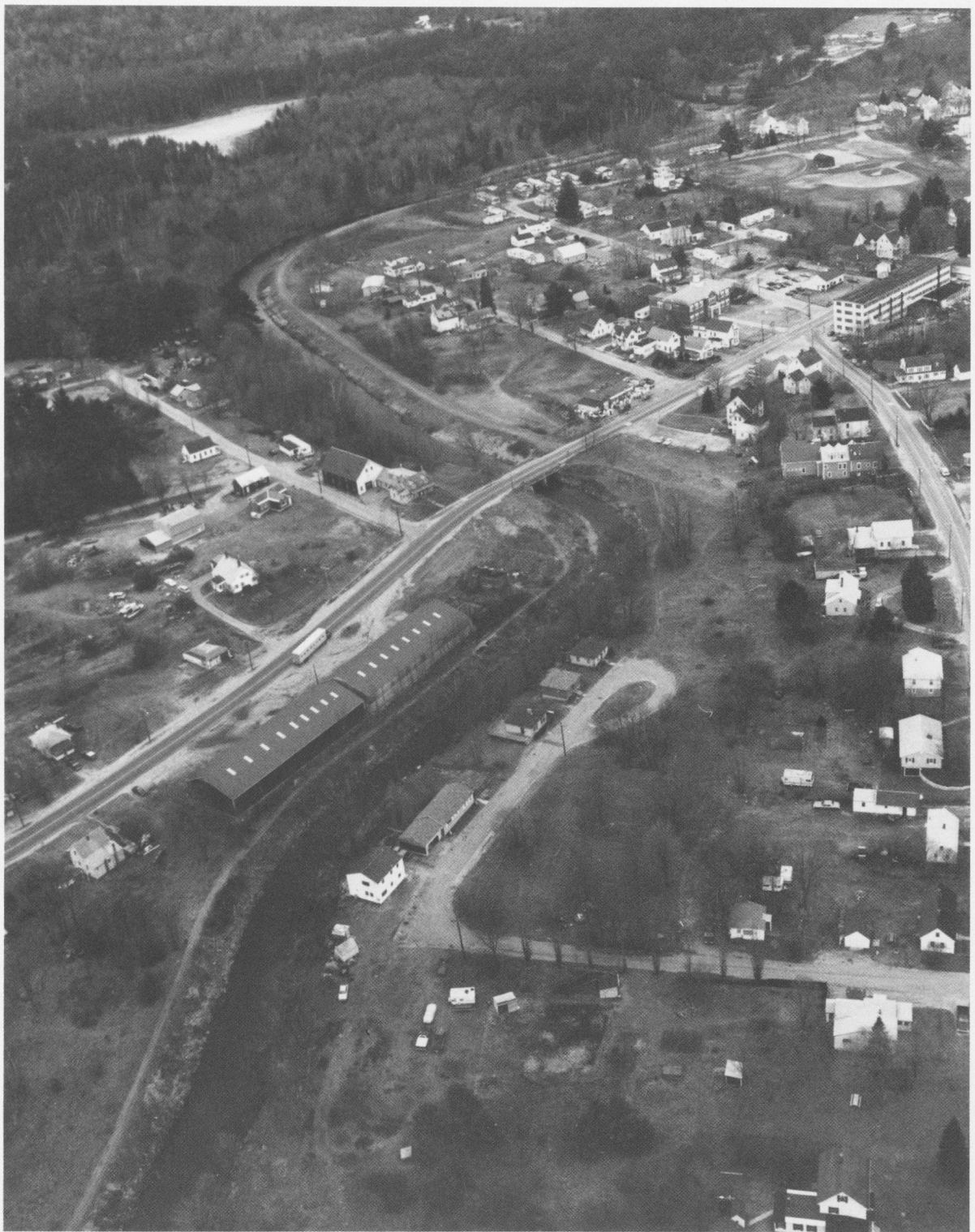
The Cocheco River Local Protection Project extends along 7800 feet of the Cocheco River and is divided into upper and lower halves by the South Main Street Bridge (center). This photo shows the entire project as it winds through Farmington.
