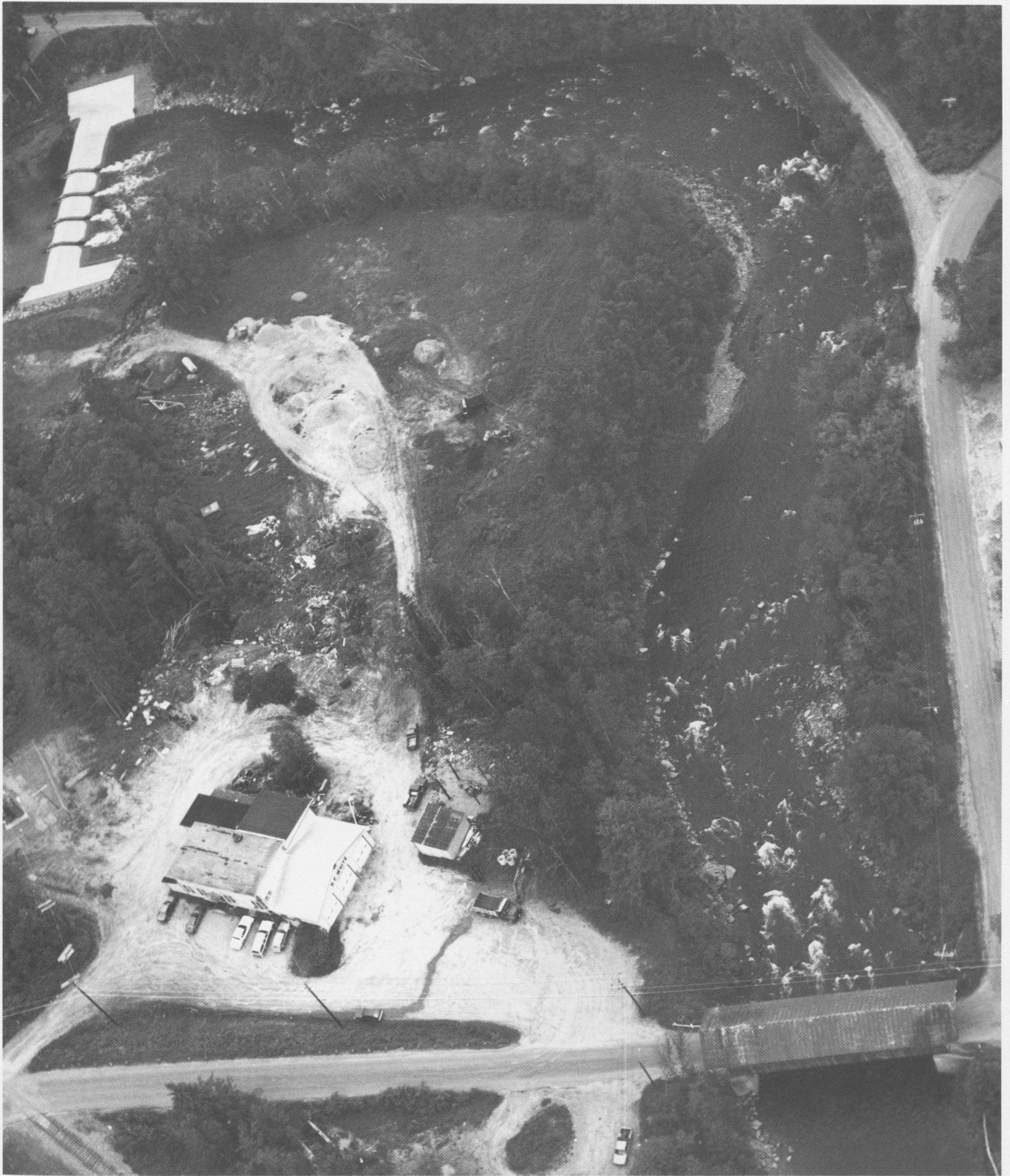
A 160-foot-long weir (top left) across the Israel River in Lancaster is designed to impound ice, reducing the threat of ice jams downstream. The project protects about 12 acres of commercial, industrial, and residential property.
