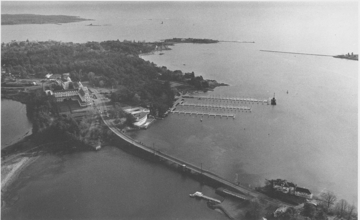
The project at Little Harbor, situated between New Castle and Rye, included the construction of a breakwater off Frost Point (right); a breakwater off Jaffrey Point (left of the Frost Point breakwater); and an entrance channel leading up to the Bascule Bridge (bottom).
