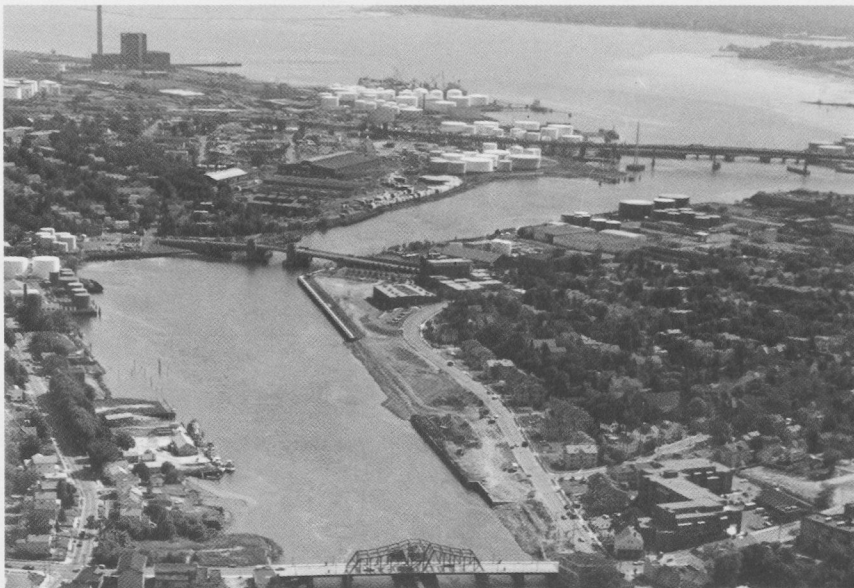
The three breakwaters (above) at New Haven Harbor in New Haven, Connecticut, help protect the harbor (left) from storm-driven winds and waves.
