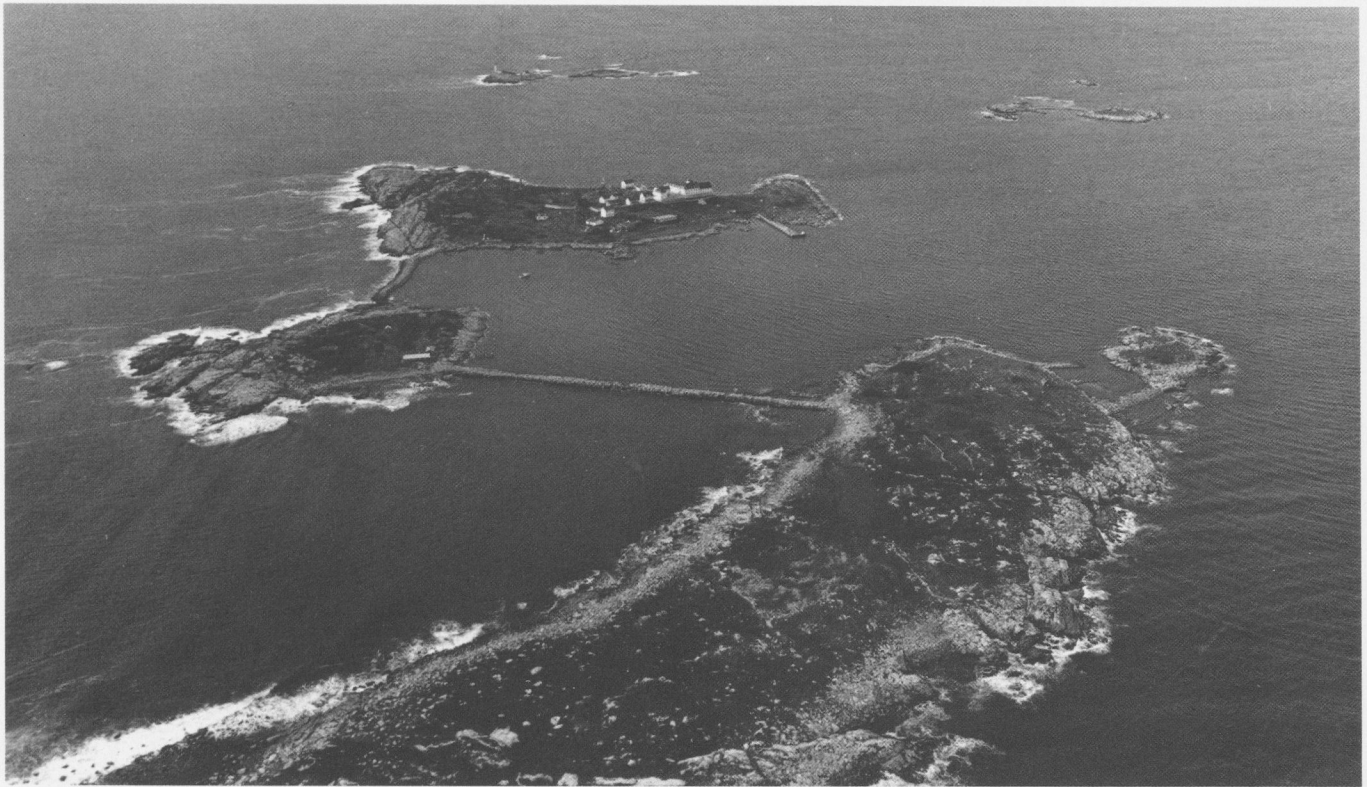
The three breakwaters at the Isles of Shoals form Gosport Harbor, in the center of the photo. The first breakwater connects Malaga Island, the small island at the far right, with the much larger Smuttynose Island; a second breakwater extends from Smuttynose Island across to Cedar Island (middle of photo); and the third breakwater connects Cedar Island with Star Island.
