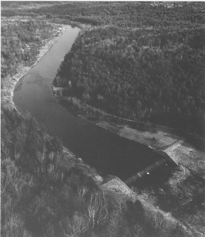
Canal II (both photos) connects the flood storage area behind the dam at Hopkinton Lake with the flood storage area behind the dam at Everett Lake, allowing the dams to function as a single unit. Canal II is a 10,400-foot-long strait, of which the upper 2000 feet is Drew Lake (top). Floodwaters pass from Elm Brook Pool behind the dam at Hopkinton Lake to Drew Lake/Canal II. These floodwaters then flow down the canal and empty into the flood storage area behind the dam at Everett Lake. The bottom photo shows the end of Canal II as it empties into the Everett Lake flood storage area.
