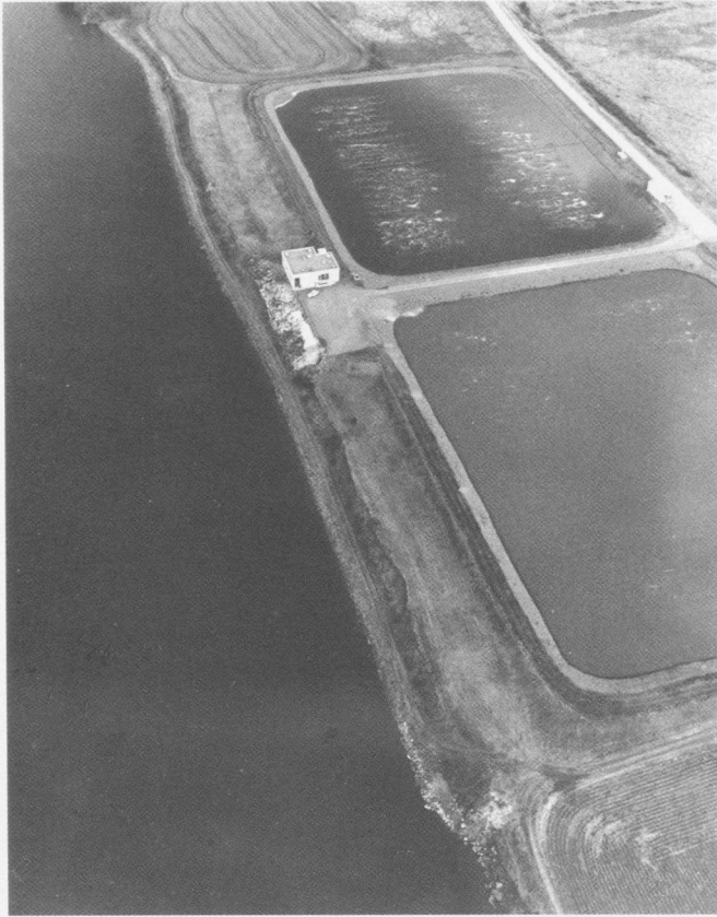
The 1300 feet of stone slope protection along the Connecticut River in Charlestown protects the town's wastewater treatment facility (center).
