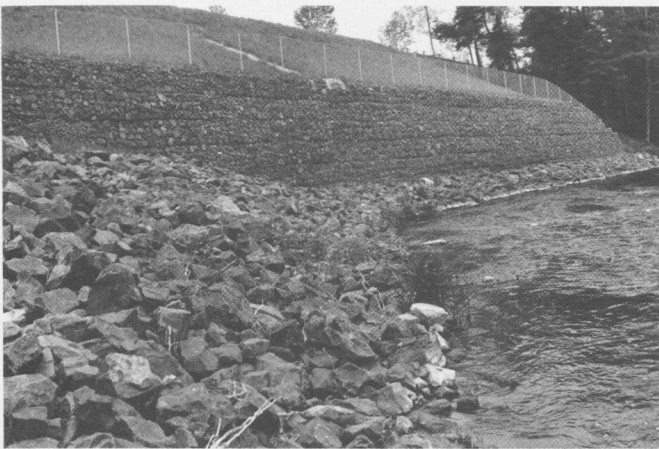
The retaining wall on the Nonnewaug River in Woodbury, Connecticut (left) is made of gabion, or wire mesh baskets filled with stone. The right photo shows gabion in closer detail.
