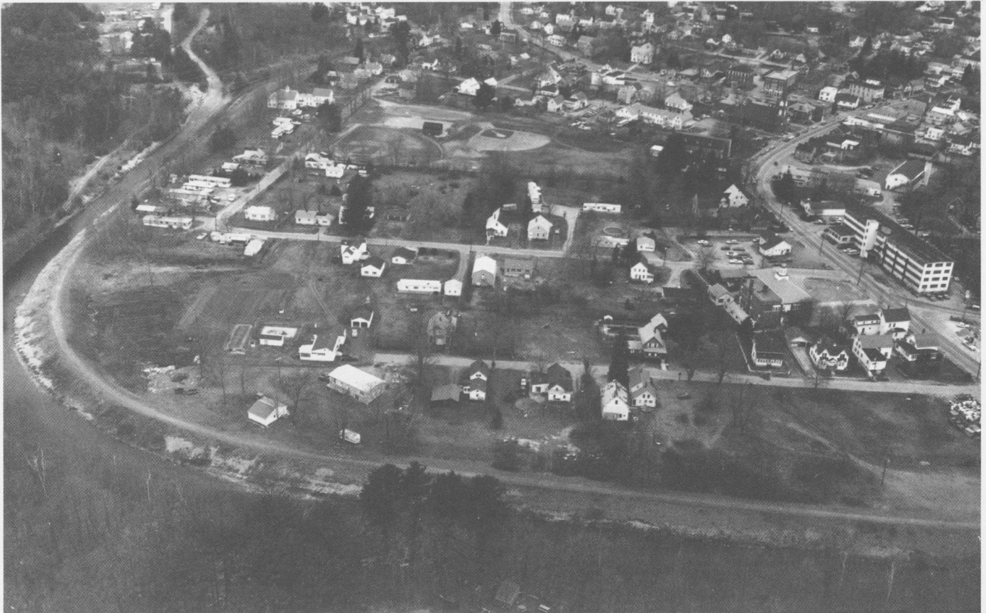
The upper half of the project begins near the confluence of the Mad and Cocheco Rivers (top left) and involved constructing 3000 feet of dike along the left bank of the river, and enlarging and straightening about 3100 feet of the river channel.
