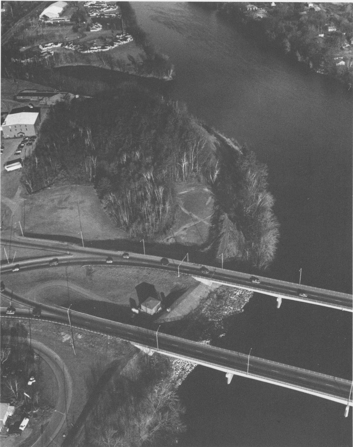
One of the features of the Nashua Local Protection Project is a 3025-foot-long dike that helps protect 70 acres of industrial and residential property. The dike starts along the right bank of the Nashua River (top left). After the Nashua River joins the Merrimack River, the dike continues along the Merrimack River before ending several hundred feet past Route 111 (center). While much of the dike is hidden under brush, a section of dike with stone slope protection can be seen between the north and south overpasses of Route 111. The structure behind this section of dike is the pumping station.
