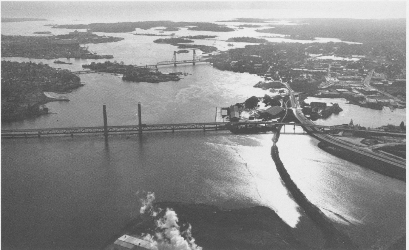
Portsmouth Harbor. The 6.2-mile-long channel, 35 feet deep and generally 400 feet wide, was widened by removing ledge in its bends, including one at Badgers Island, just left of center in the photo.
