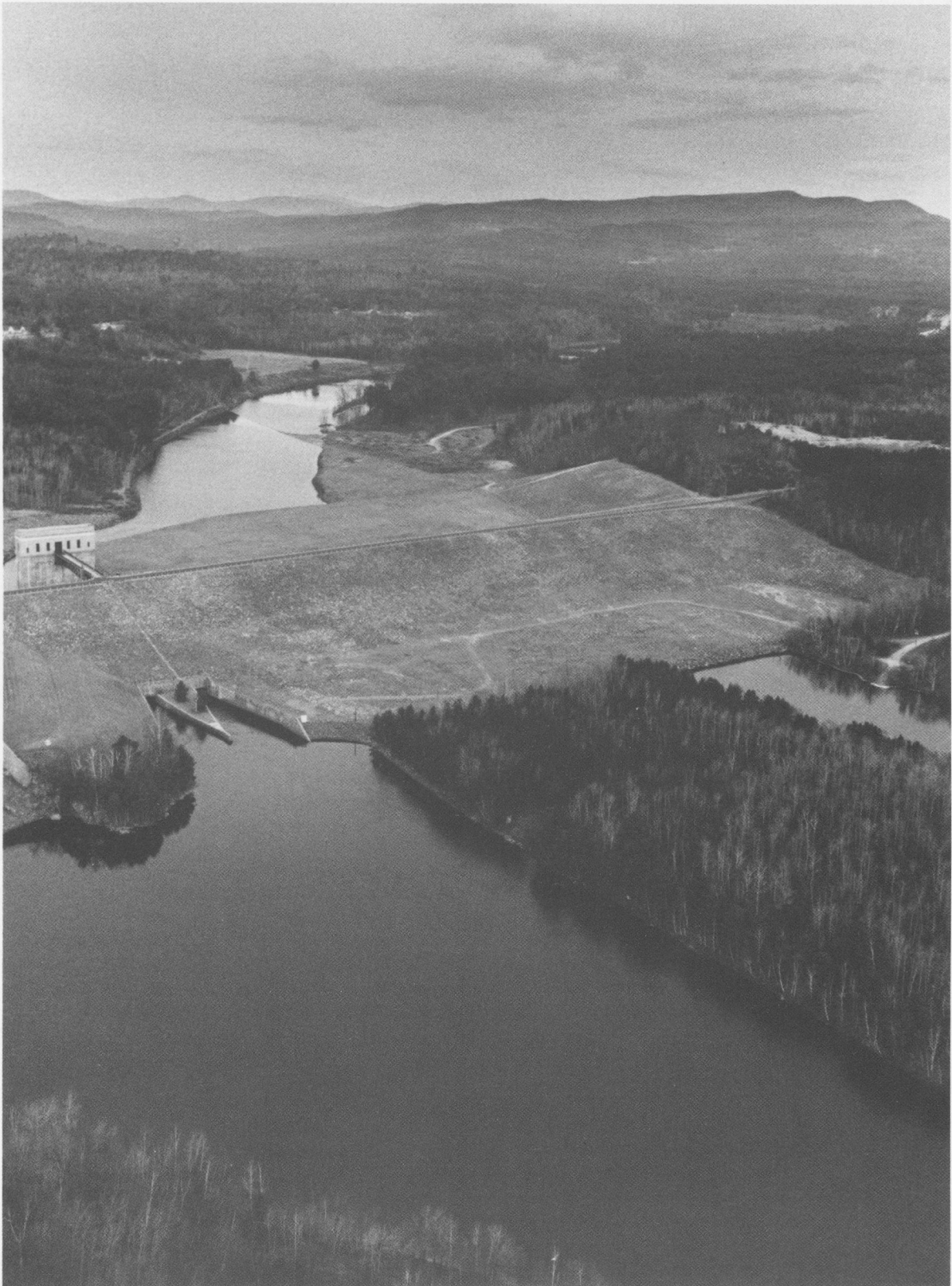
Franklin Falls Dam
