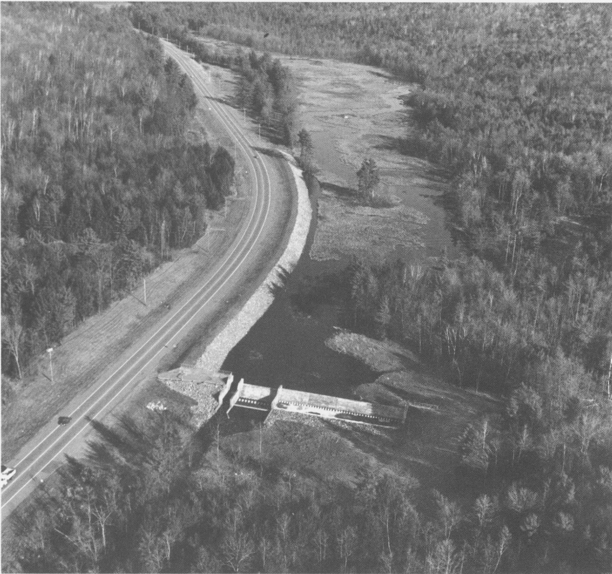
Completed only in 1986, the Beaver Brook project in Keene has already prevented an estimated $1.6 million in flood damages. The project includes a 250-foot-long concrete dam across Three Mile Swamp (center) and a 1100-foot-long dike that runs parallel to Route 10 (left).
