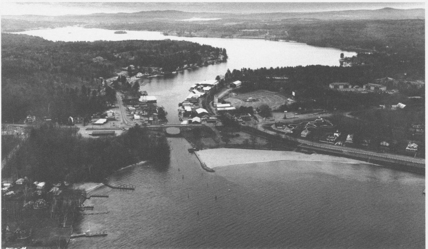
The project at Lake Winnepesaukee in Laconia consists of a navigable passageway through Weirs Channel (center). Weirs Channel connects Meredith Bay (bottom) with Paugus Bay (top).
